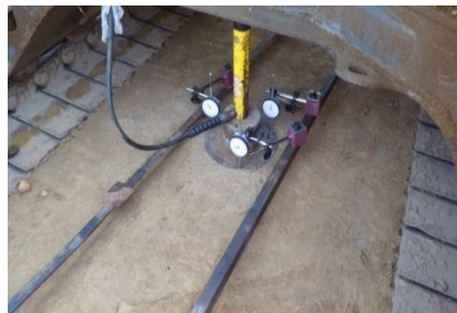
Figure – 02: Prepared arrangement of Plate Load Test (PLT)
